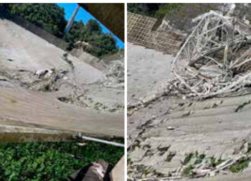
AFTER THE FALL. The steel carcass of the receiving platform and an access platform lie in a tangled heap across the remains of the reflector dish. UCF
